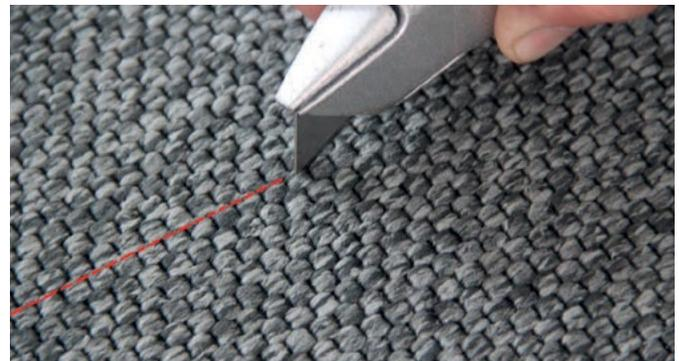
*Cut the edges with a sharp trapezoidal knife. Change the blade of the knife regularly. When cutting, it can be helpful to hold the knife at a slight angle to give a smooth cut.*
