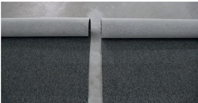
*We recommend fitting the carpet in all rooms or levels in one direction only, due to the clearly visible texture of flatwoven carpet.*
