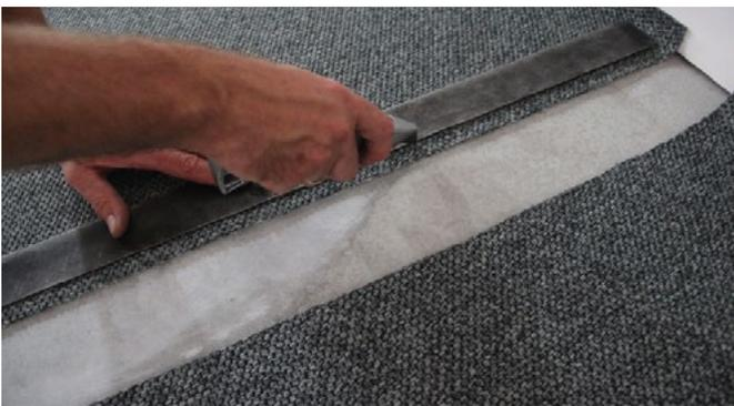
*Cut the final edges following the straight warp binding yarn.*
